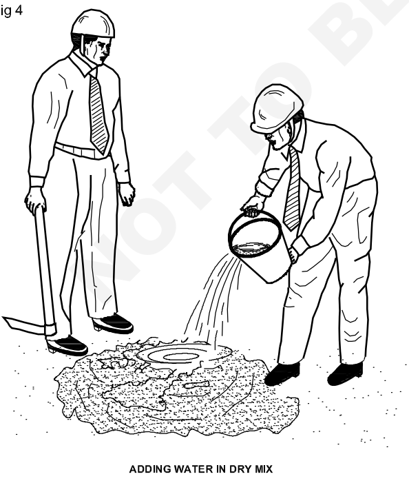
DRY MIXING OF CEMENT AND SAND
